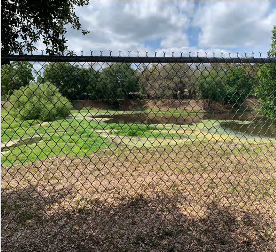
Example of a fenced stormwater pond along 22nd Street across from Middleton High School
